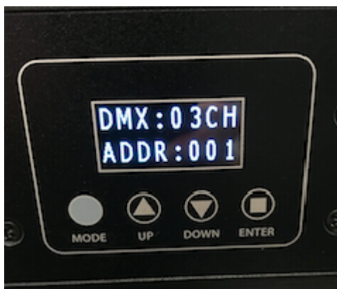
DMX CABLE CONNECTED
