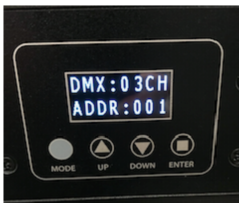
DMX CABLE CONNECTED
